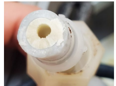
Figure 3-2. Scale Accumulation in Tubing
