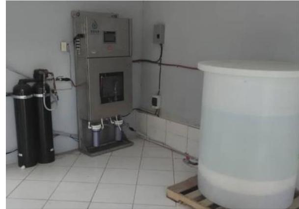
K Series are electrolytic systems that uses salt, electricity (AC) and water to produce a hypochlorite-based mixed-oxidant solution—liquid chlorine—that maintains its strength for two to three weeks without stabilization.
